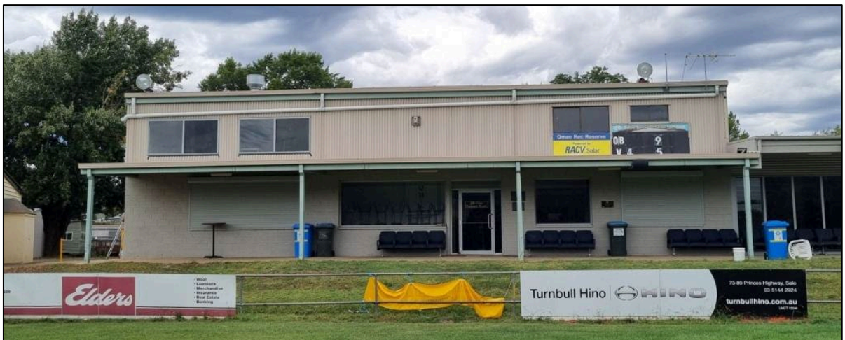
Omeo accommodation building.
